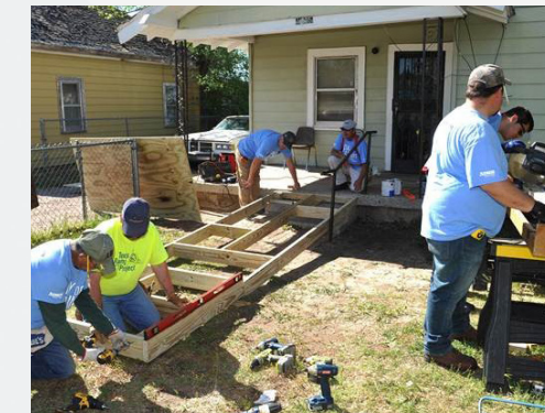
A Pantex volunteer team builds a wheelchair ramp for the Texas Ramp Project during the Amarillo and Canyon Day of Caring.
